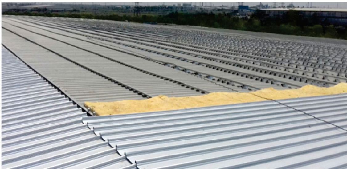
Variable Spacer brackets on top of LYSGAHT TRIMDEK® Liner profile.
