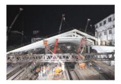
including rafters, bracings, strut tubes was done by handling them in the air with multi-crane system. The fixing was done with the help of boom lifters, which carried men and material to bolt the joints. Work for fixing of Z-section pre-punched and pre-galvanised purlins over erected rafters was also done in parallel, to save the time in the same blocks. The entire work was done in power-blocks without any slewing or lowering of overhead electric lines.
